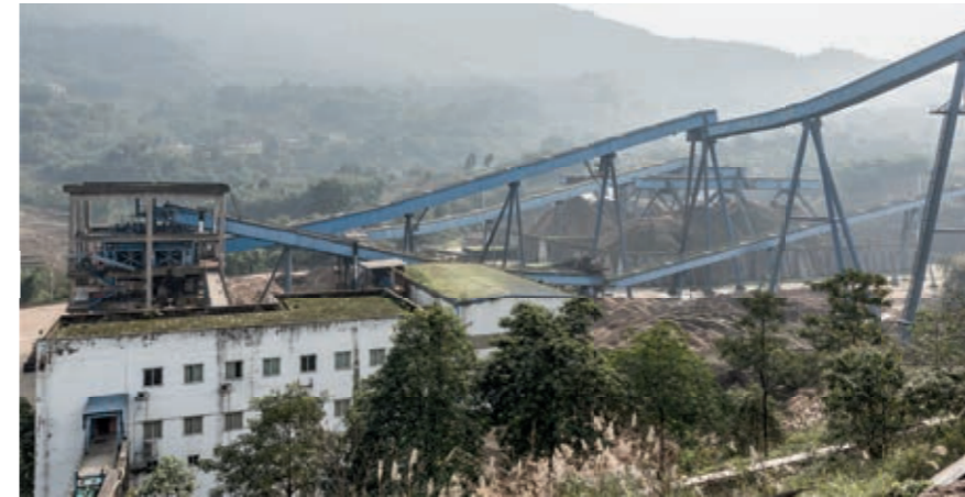
The fully integrated mill makes tissue using bamboo as its main source of fiber. ANDRITZ also supplied the original fiberline.
